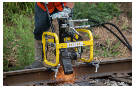
Grinding with head wash grinder.
